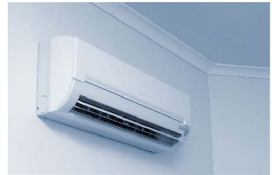
Clearance from ceiling and easy access for maintenance
