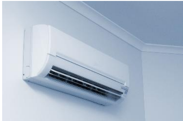
Indoor units located more than 30 cm below the ceiling (best practice 30-45 cm from ceiling)
