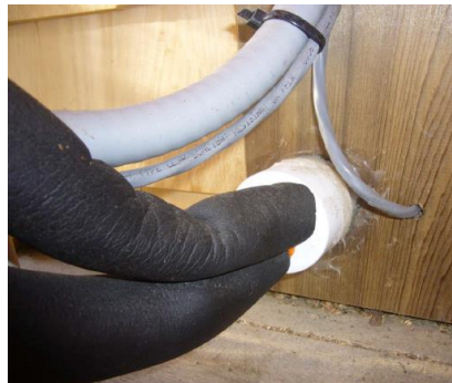
Envelope penetration properly sealed
